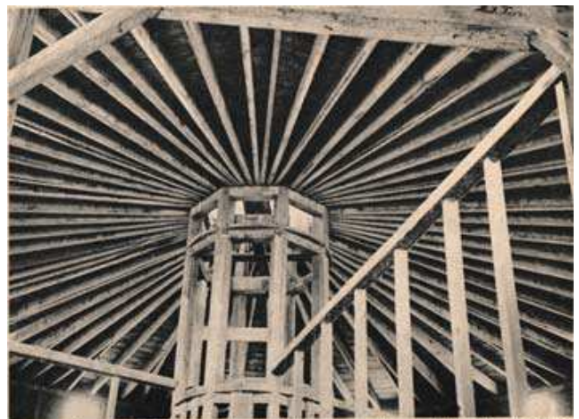
This interesting view of the interior of the village's famous round barn, a Berkshire landmark since 1826, shows the architectural skill with which Shaker craftsmen were gifted. This intricate network of hand-ched beams has supported the roof of the building for nearly 150 years.
